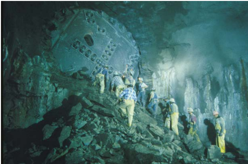
A tunnel boring machine is “daylighting” as it completes one of the initial TARP deep tunnel bores.
