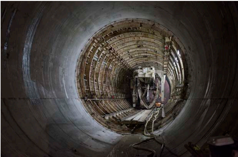
A segment of deep tunnel is lined with concrete, while the process of placing the forms for the next tunnel segment awaits a concrete pour and liner.
