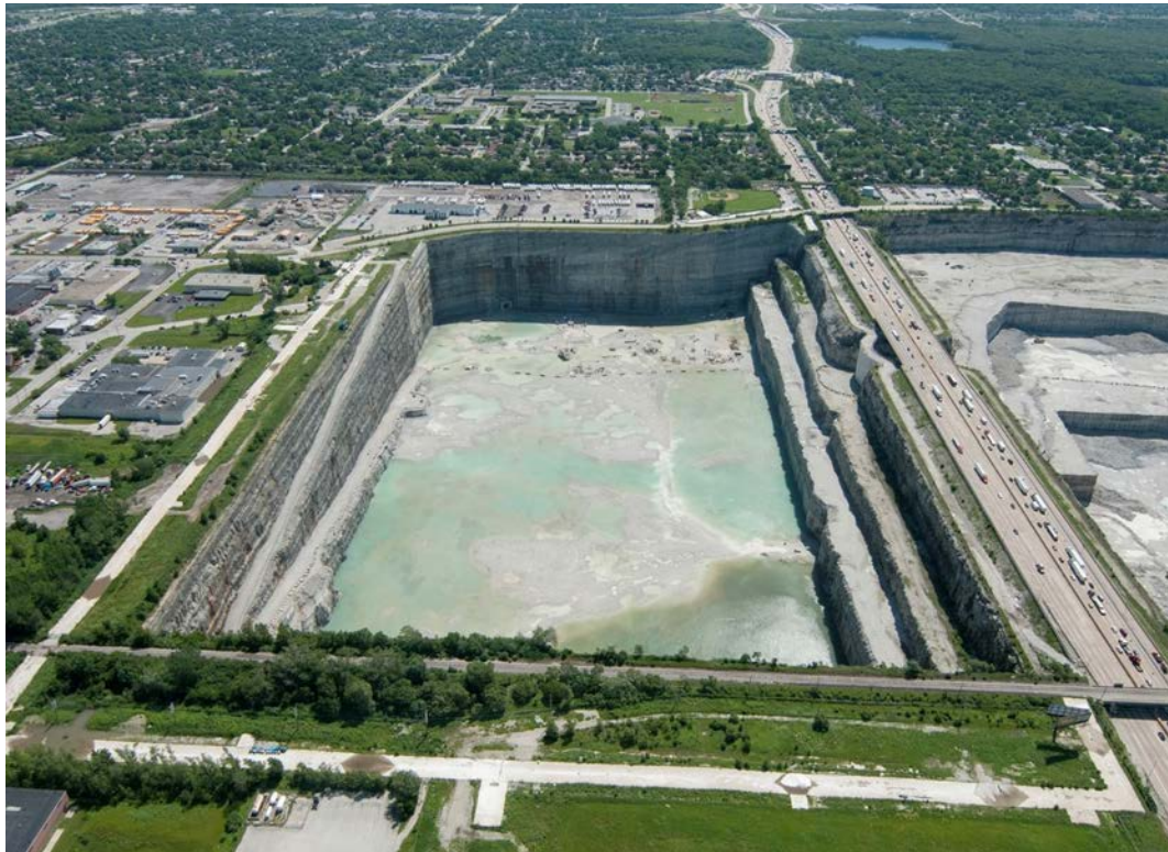
Viewed to the east, Thornton Composite Reservoir measures 300 feet deep, one half mile long, and approximately one third of a mile wide, with a capacity of 7.9 billion gallons of combined sewer overflow and floodwater storage.
