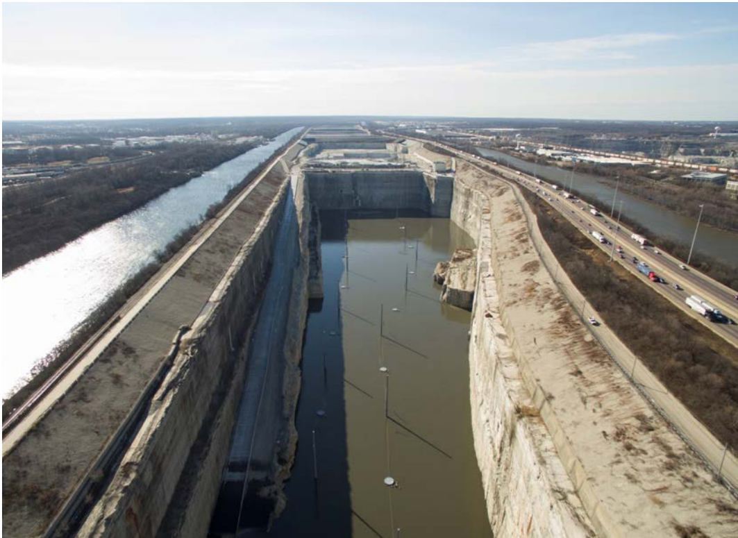
McCook Reservoir Stage 1 takes on water to protect 37 communities while surrounded by the Chicago Sanitary and Ship Canal (left), Interstate 55 (Stevenson Expressway), the Des Plaines River (right), and the McCook Reservoir Stage 2 to the southwest, which is under construction.
