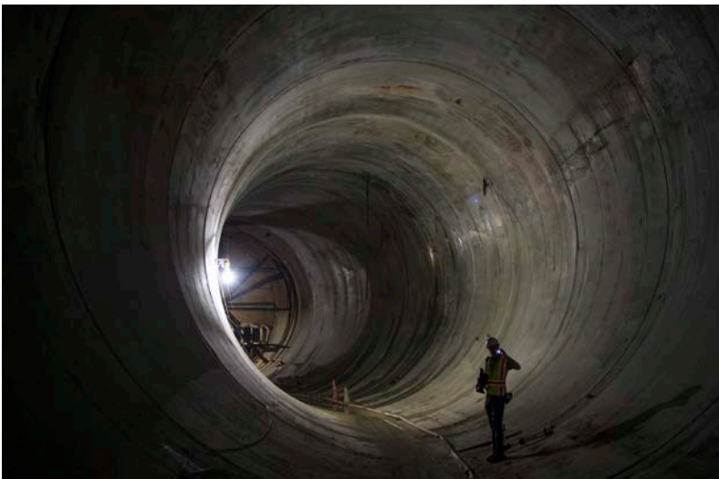
A segment of deep tunnel is lined with concrete, while the process of placing the forms for the next tunnel segment awaits a concrete pour and liner.
