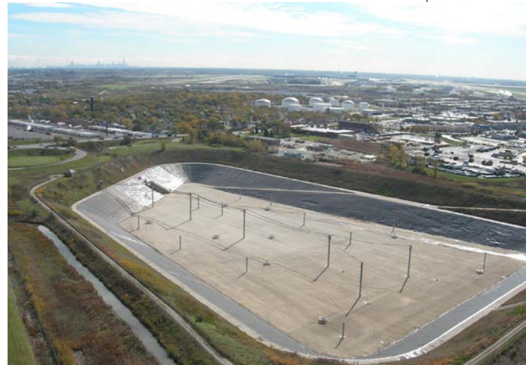
The Majewski Reservoir contains up to 350 million gallons of combined sewer overflow water and serves the TARP Upper Des Plaines Tunnel System. The downtown Chicago skyline to the southeast is visible in the background.
