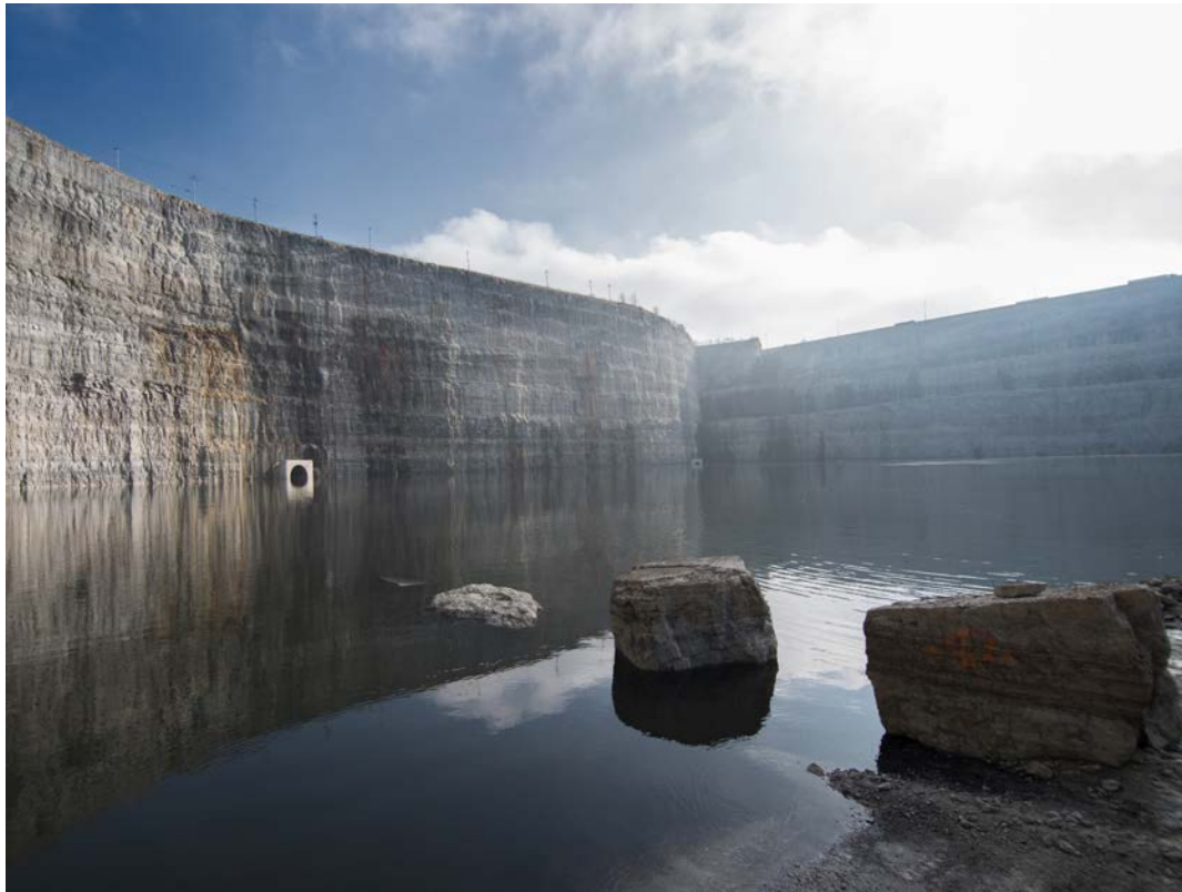
Water surfaces inside the Thornton Composite Reservoir, while the 300-foot-tall reservoir highwall and portal to the Calumet Tunnel System appear in the background.
